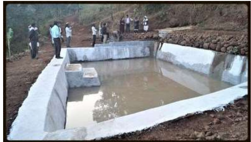
A water storage tank constructed at Sarodhadadar, Kabirdham to collect spring water for drinking purpose
